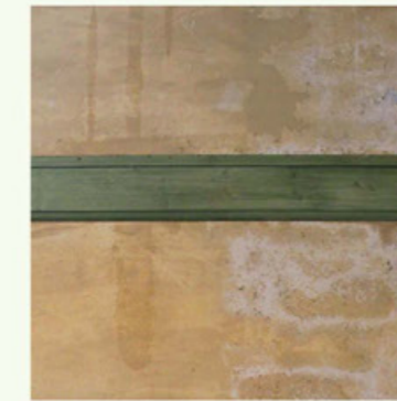
2. Wooden slat on wall inside
