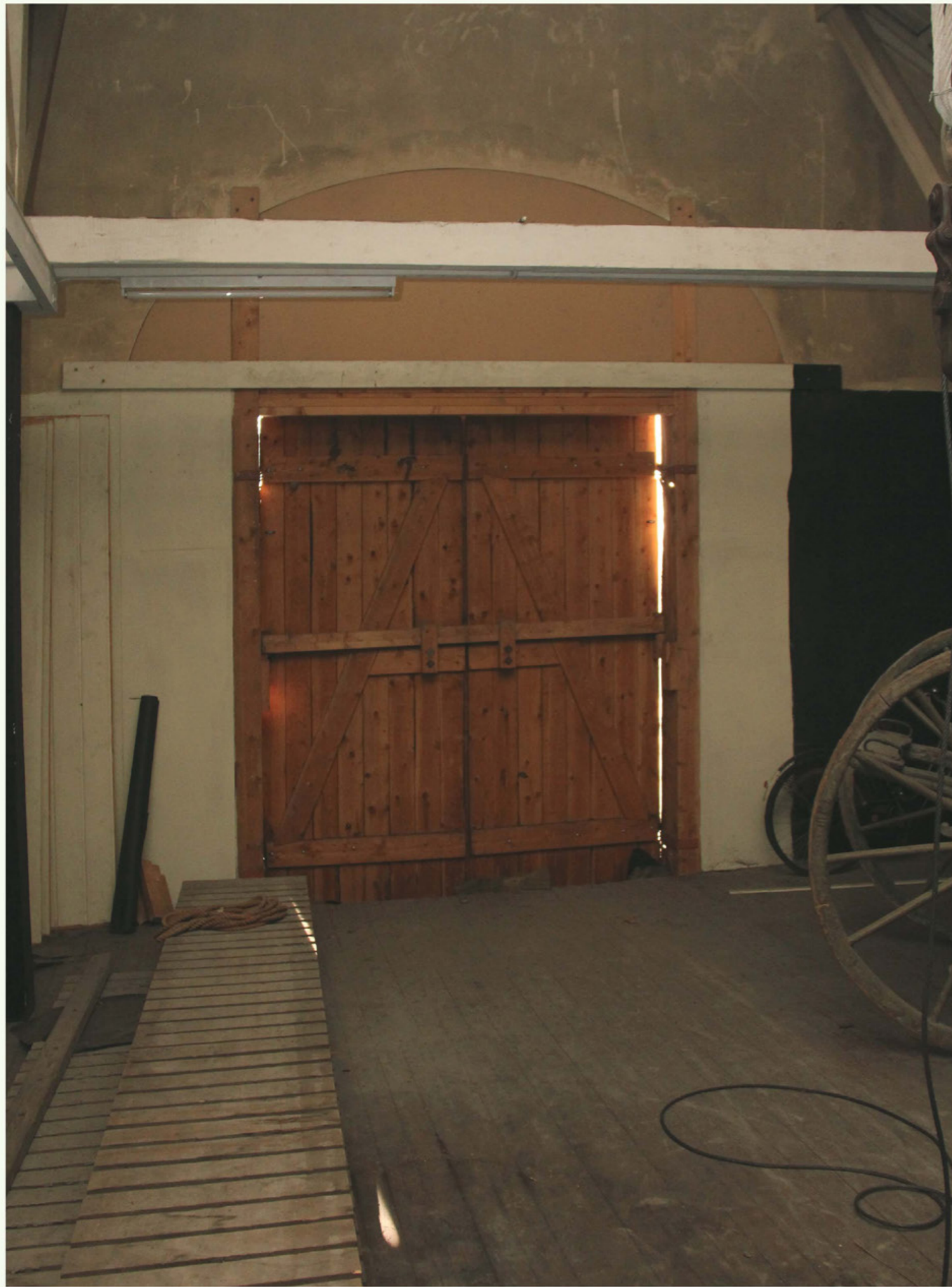
Doors in the southern wall on the 1st floor, that can be opened to move bigger objects in and out of the space
