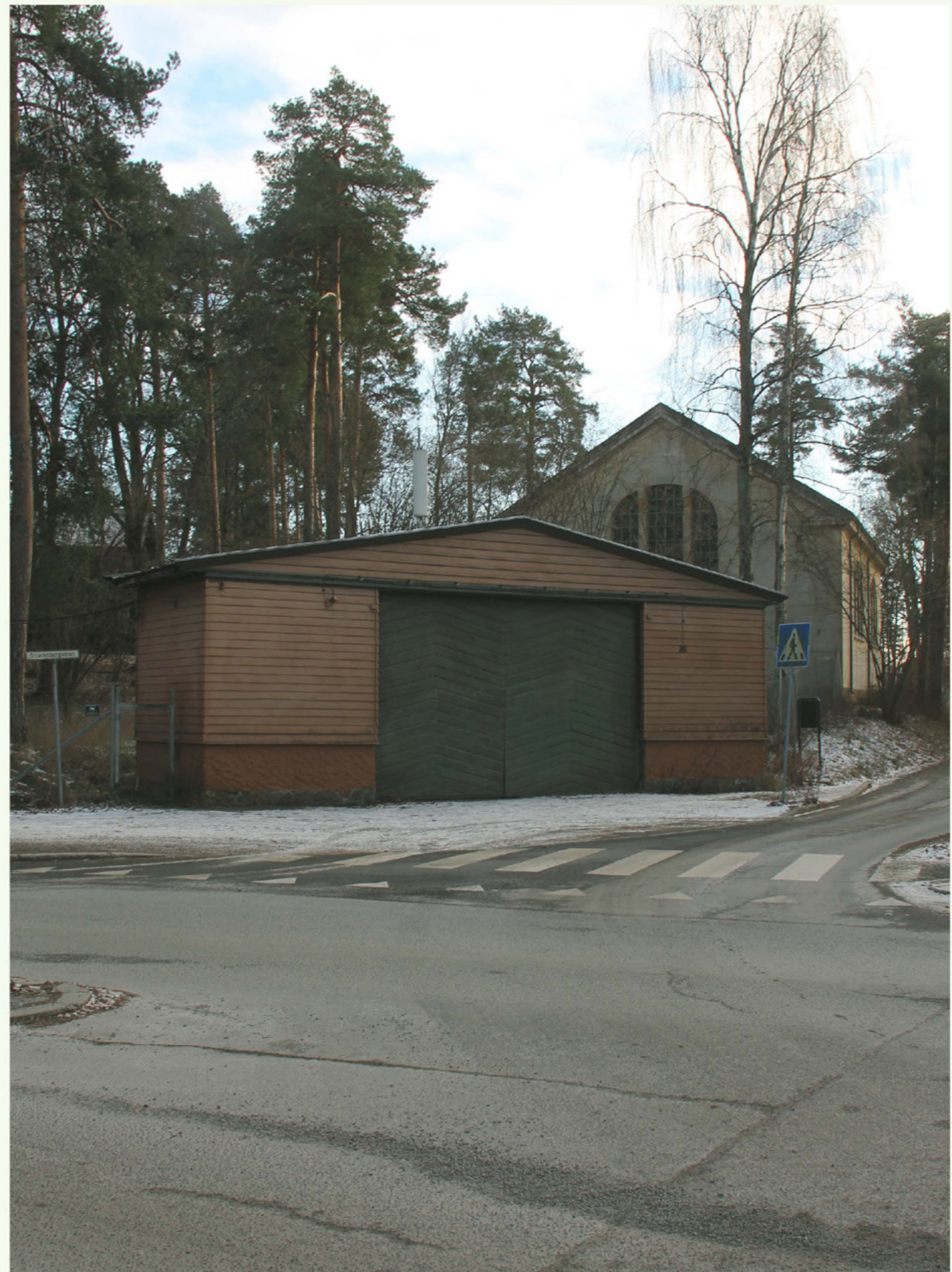
The gate seen from the street. This gate is currently it is not in use
