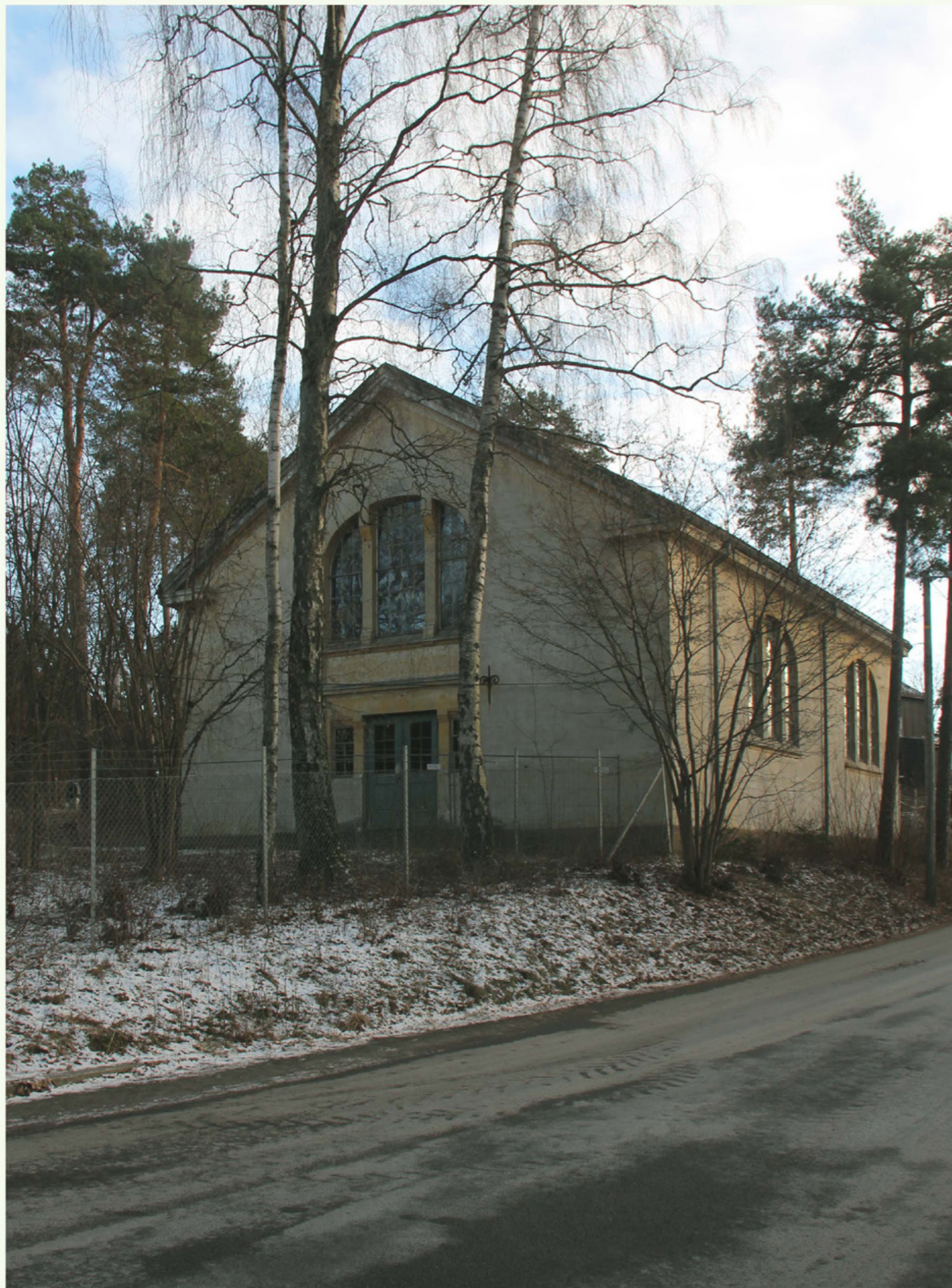
The northern facade of Vognhuset seen from the street
