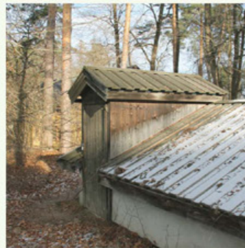
11. Shed with technical room
