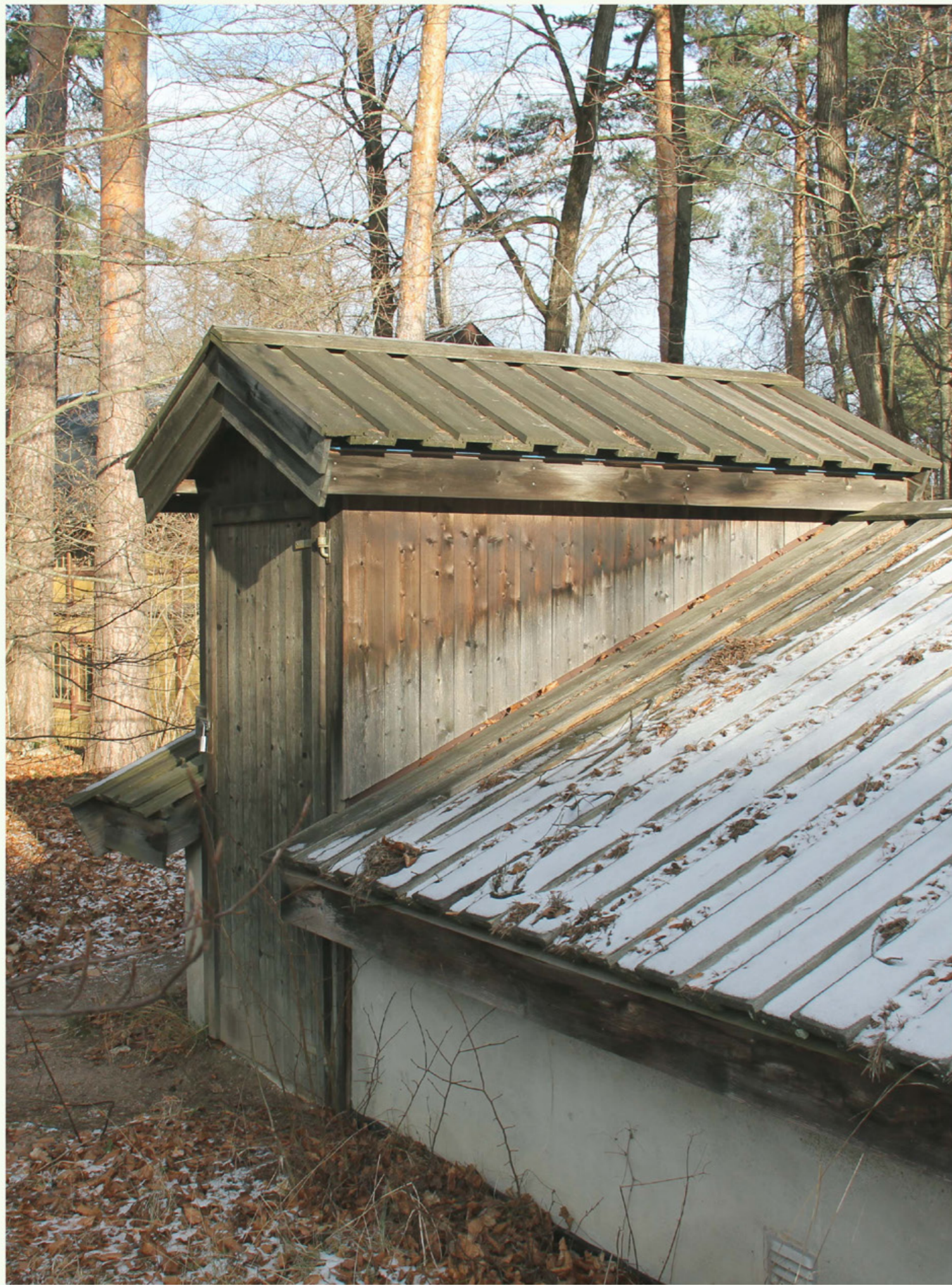
Shed with technical room
