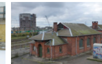
Vestre Pumpestation Vesterbro, 1901, Ludvig Fenger In use for cultural events
