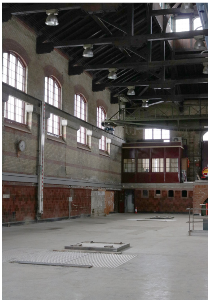
The now empty main hall, formerly containing the spill water pumps. On the floor you can see the old podiums where the pump engines used to stand.
