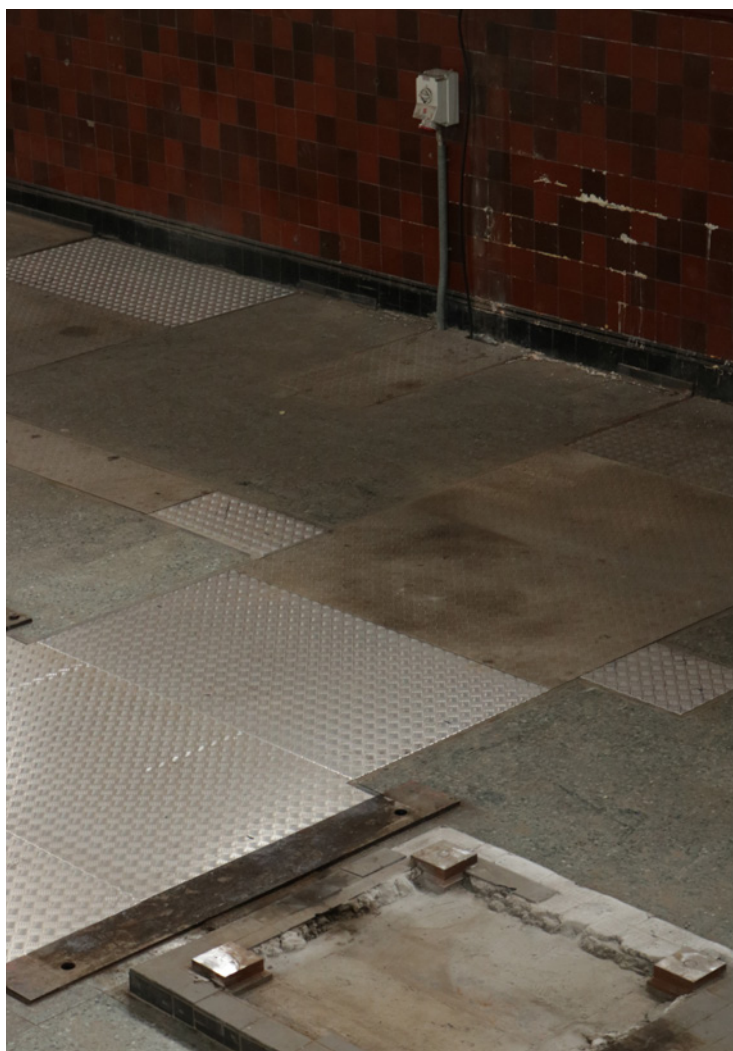
Metal inlays in the terazzo floor and the old machine podium - Traces from former use.
