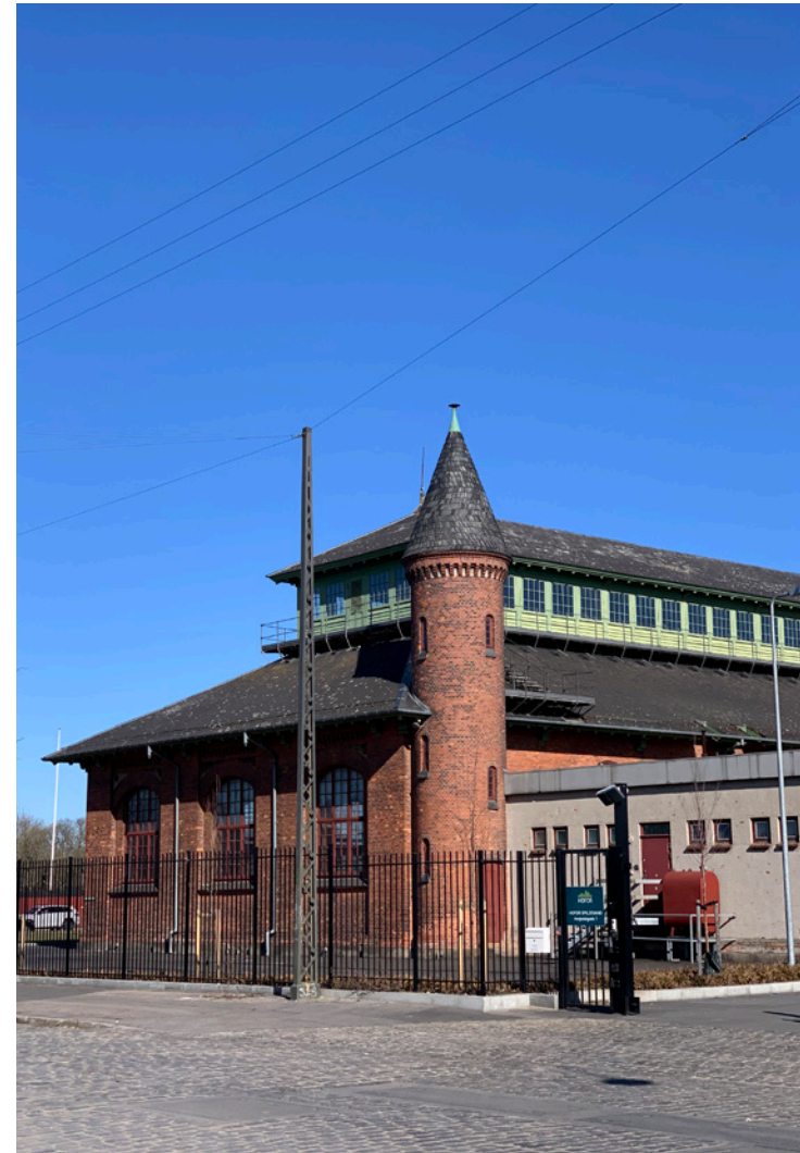
The pump station seen from Herjedalsgade. In the front to the right you see the access road through the tall fence. To the right you see the grey side building, an original, but heavy transformed building.
