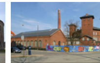
Kloakpumpestation Østerbro, 1894, Ludvig Fenger In use as a youth club
