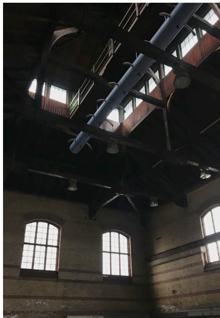
The characteristic roof construction
