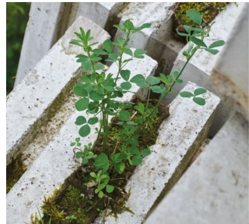
Figure 3.13: Small folds in concrete to support insect habitats (Weiner, E. Stevens, P. 2015)
