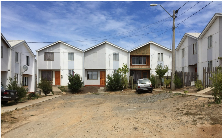
Villa Verde Housing by Elemental °
