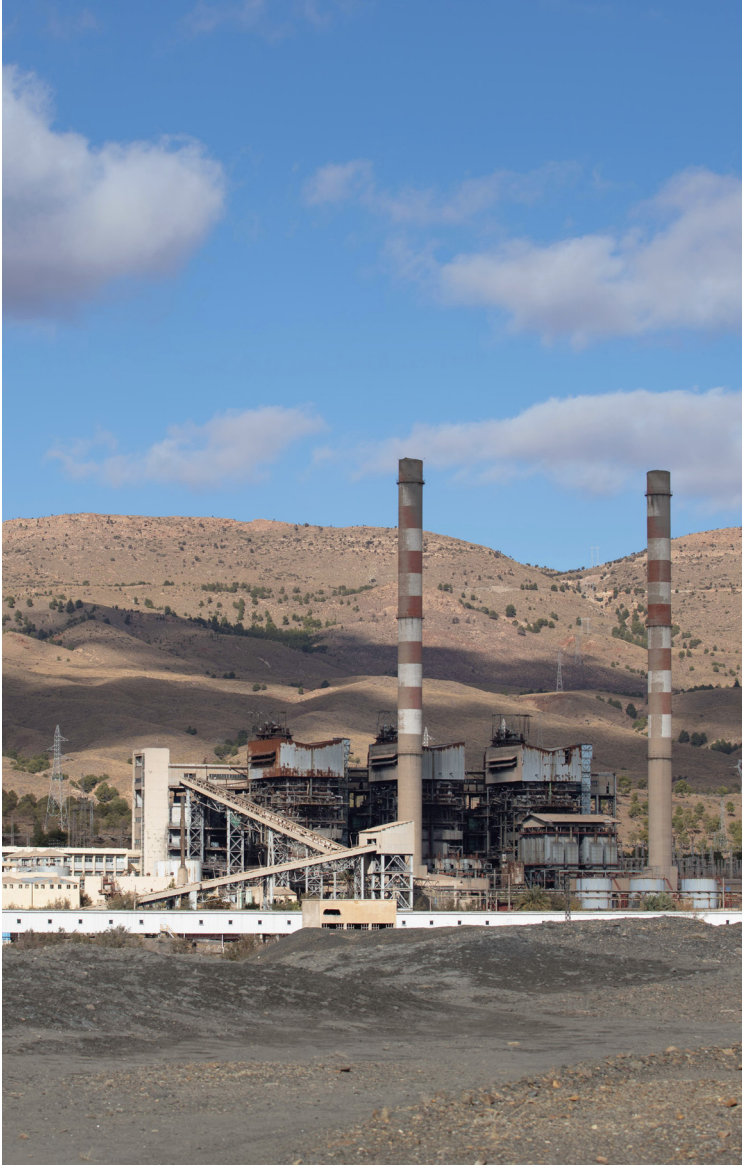
The abandoned coal power plant currently on my intended site
