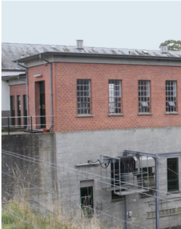
“Den nye pumpestation”, 94m 2 (1939)
