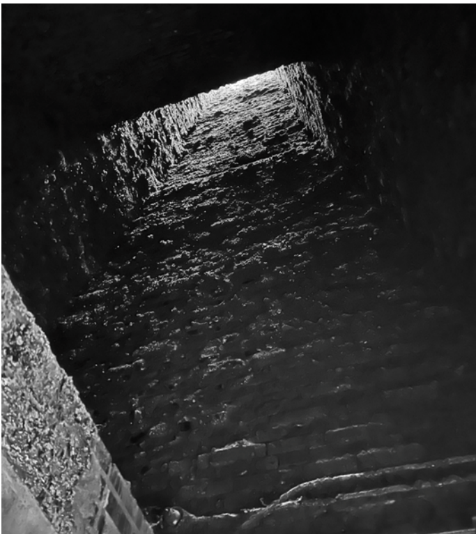
View inside chimney
