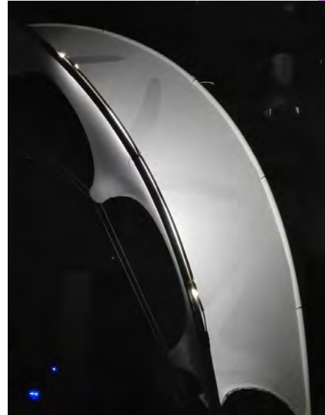
F 2.37: Star-shaped knit material specifications of differentiated knit structures in Isoropia tensile unit, using Graded Fields approach. CITA 2018
