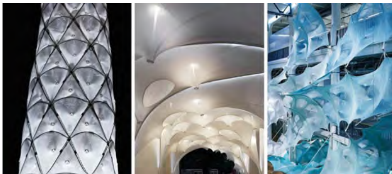
Fig. 2 Large-scale structures, employing CNC-knitted textile as a structural membrane. Left to right: Hybrid Tower 2016, Isoropia 2018, Zoirotia 2021. Authored by
