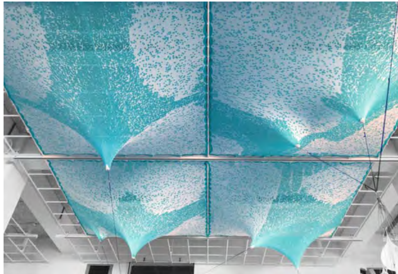
Fig. 18 The CNC-knitted textile panels design with angles loading directions demonstrates the benefits of using tensioned-based material differentiation strategy
