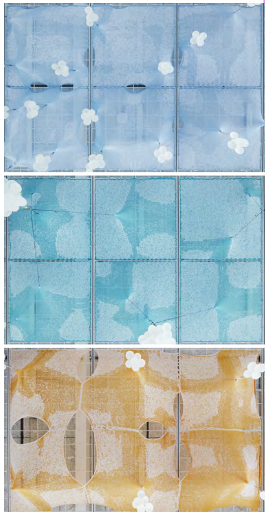
F 3.25: GraCe knitted ceiling panels, where the form of textile strain shapes the knitting pattern. Sinke 2022, Photo A. Ingvartsen
