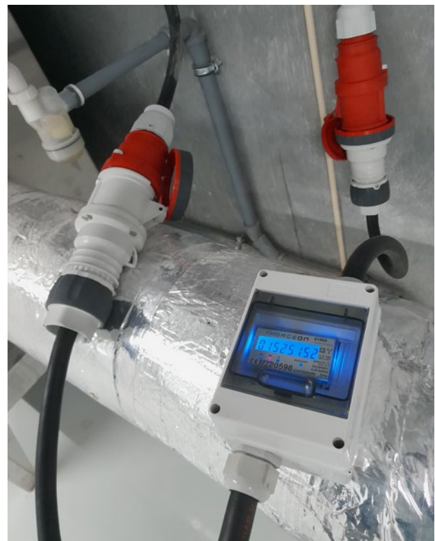
Mobile energy meter mounted directly on the dehumidifier.
