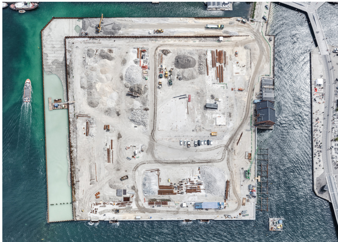
Papirøen as a construction site, © Cobe
