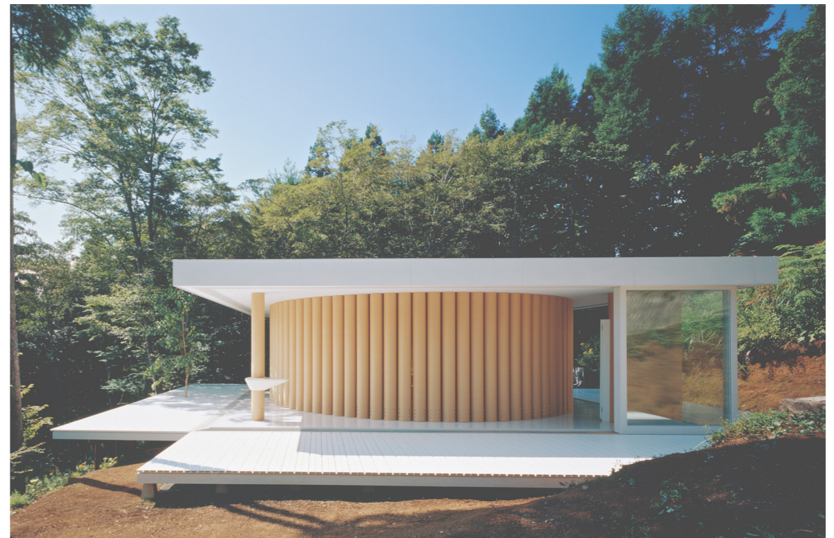
Shigeru Ban, Paper House This was the first project in which paper tubes were authorized for use as a structural basis in a permanent building.
