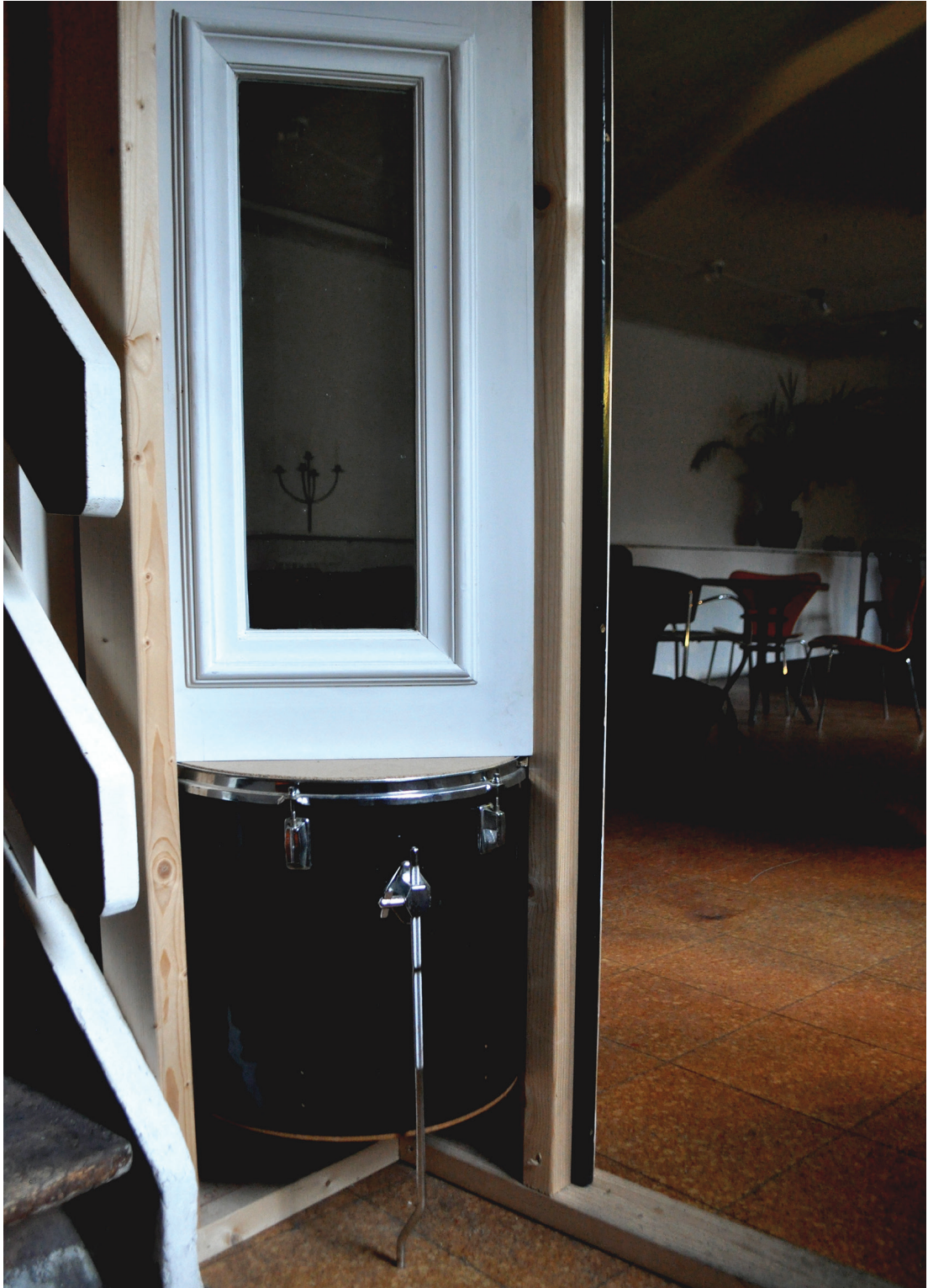
Stair way between the shared kitchen, and the exhibition room A drum used as support in a room deviding wall piece made of a reclaimed window.
