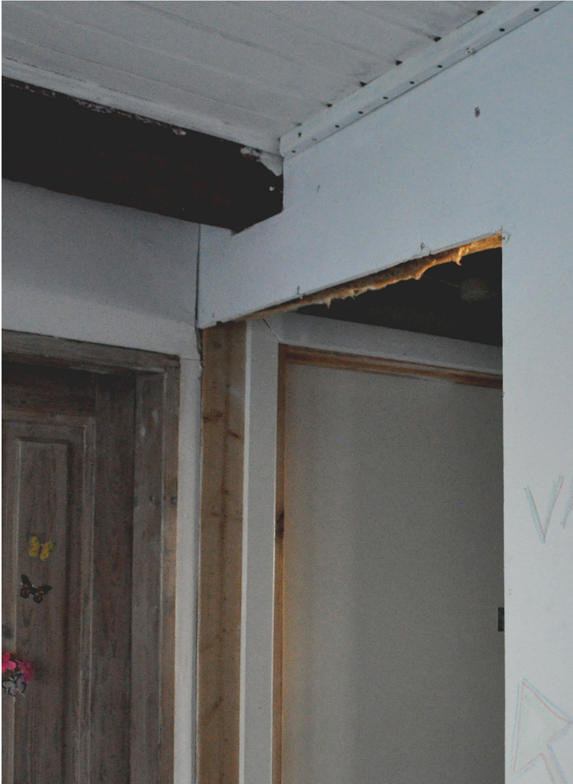
Self made plaster walls
