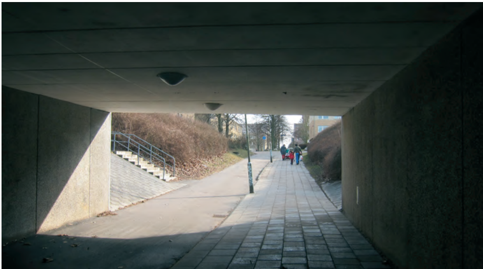
Figure 2.19. Tunnel exit/entrance in Holma, (130414). Photo by the author.
